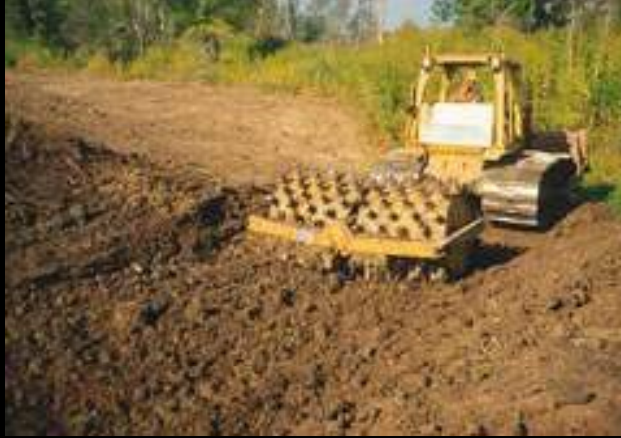
Sheepsfoot Roller to Compact Clay Soils
